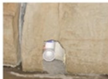
Connect plumbing at back of base piece. Hide pipe with long hollow piece (cut to fit.)
