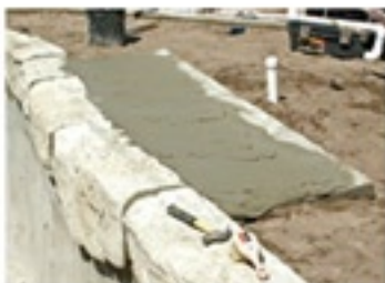
Waterfall pad for 3 Ft. Modular should be 7 feet wide, 30" front to back.
