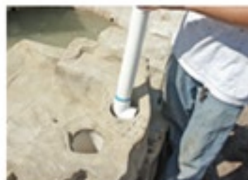
Drop plumbing sleeve in hole. Tighten threaded plug if you plan to pressure test line.
