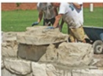
Set basin on 3/4" mortar bed. Level from left to right. Match up plumbing & concrete holes.
