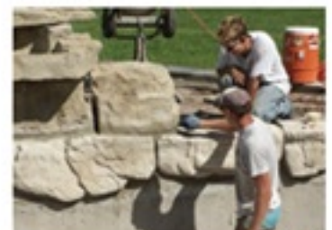
Mortar cap rocks. Clean excess mortar & rake joints about 1/2 inch.
