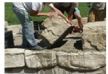
Set side boulders & mortar gap with base piece.
