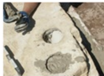
Fill concrete column with concrete.
