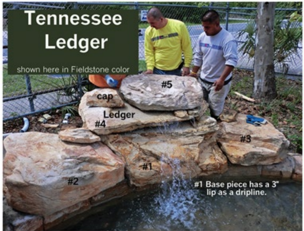
The cap rock #5 was placed on the boulder to the right in this install. Wedge piece is shown between left boulder and center base piece, not used in a radius application. The 3 large boulders and the ledger piece can be moved around as needed.
