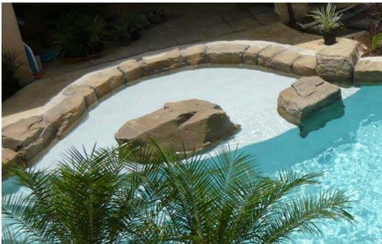
**Notched boulder look great and work well submerged in the pool on a reef step but they must be special ordered. They must either be filled with a closed cell foam or ordered as hollow boulders to be filled with concrete.**
