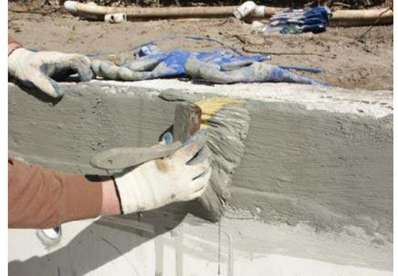
RicoRock Waterproofing is a hydraulic cement designed for fast installations:
