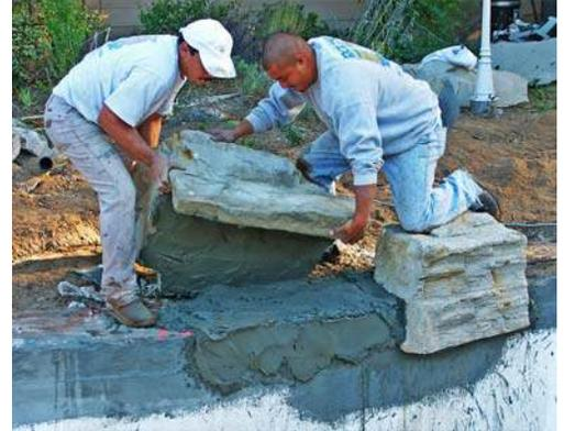
When installing on a bond beam radius there will be a gap between the boulder and the pool wall. This void should be filled with mortar, which is difficult, or with expanding foam after the mortar is set. For very large notched boulders a half inch hole can be drilled in the rock lip to inject the foam into gap between the rock and the pool wall.
