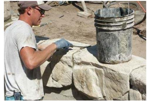
Coping/Waterline pieces should be applied after the waterline area has been waterproofed. A rich mortar should be used and the coping pieces and the contact area should each have  $\frac{1}{2}$  inch of mortar. You may need to shim up the top edge to create a 2 or 3 inch coping to match the deck height.
