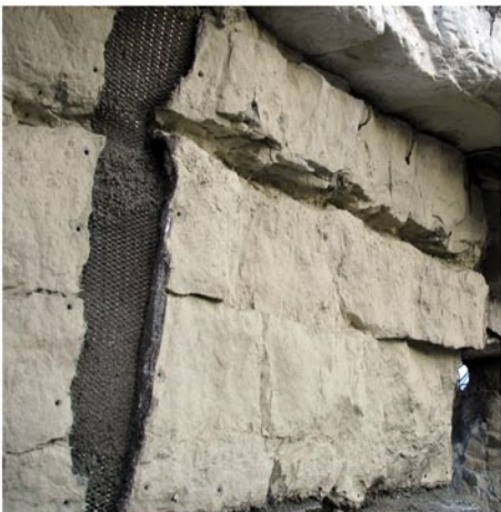
Castings are tied to rebar frame using #9 wire inserts on back of castings. Metal lathe is used between gaps. Backfill with concrete mix, protecting slide with plastic sheeting. Gaps between castings need to be hand textured.
