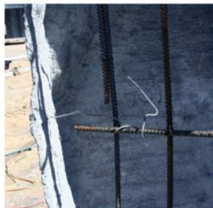
Castings are tied to rebar frame using #9 wire inserts on back of castings. Metal lathe is used between gaps. Backfill with concrete mix, protecting slide with plastic sheeting. Gaps between castings need to be hand textured.
