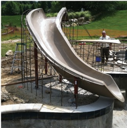
First set slide flume with steel supports from manufacturer or weld custom angle iron frame.
