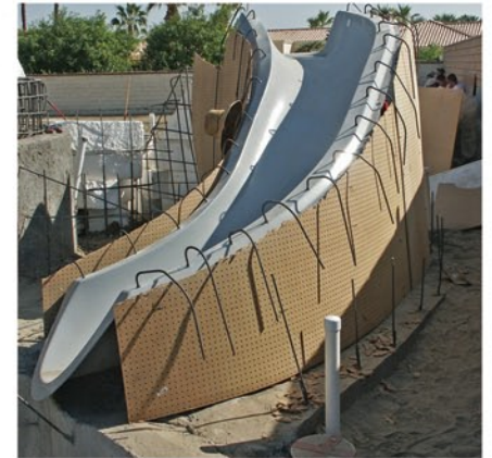
Pegboard is a good inside form for concrete backfill.
