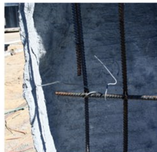
Castings are tied to rebar frame using #9 wire inserts on back of castings. Metal lathe is used between gaps. Backfill with concrete mix, protecting slide with plastic sheeting. Gaps between castings need to be hand textured.
