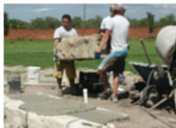
Base piece weighs 150 - 200 lbs. Use thick mortar bed.
